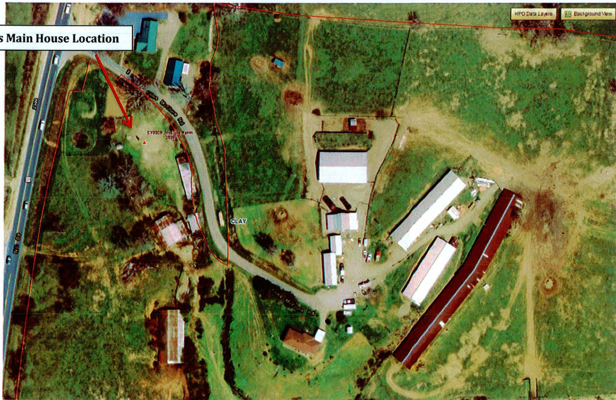
Aerial View of McClure Farm. SHPO GIS.
