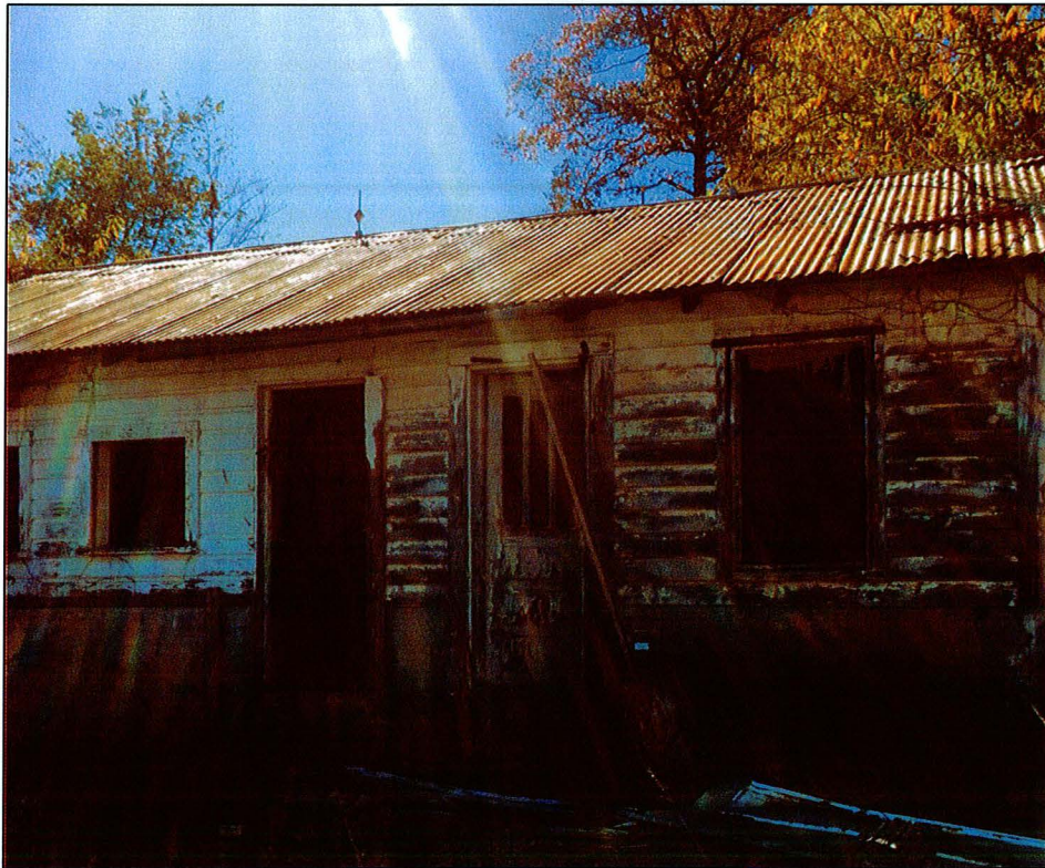
Dairy Shed, South side of Cline McClure Road, looking west. 2016
