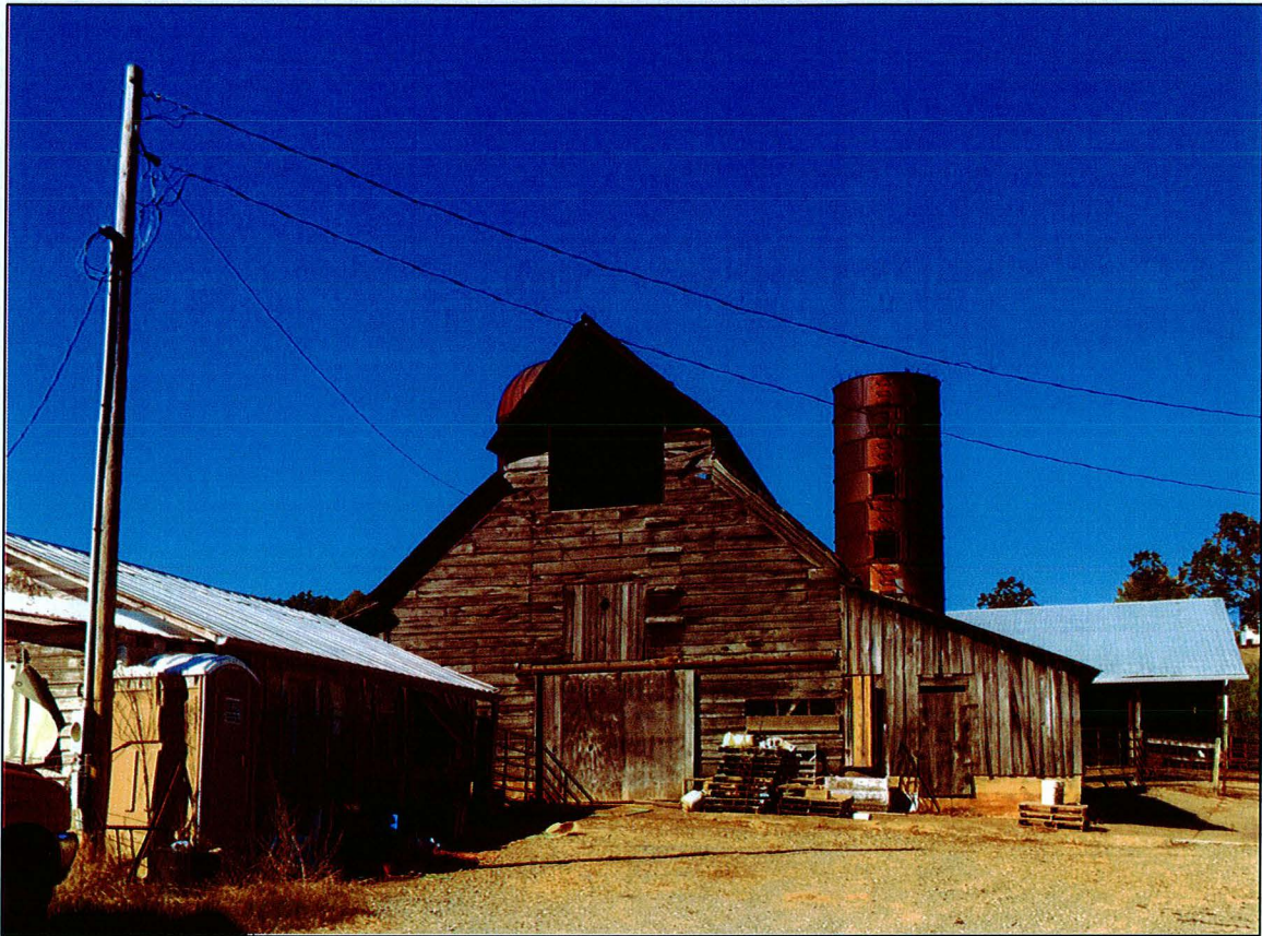
Barn, McClure Farm, looking north. 2016
